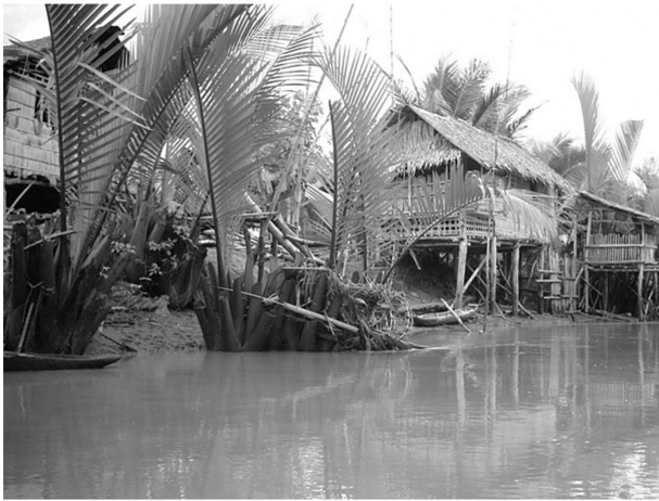
FIGURE 4 Philippine fishing villages then and now. Despite government claims that Philippine fishing villages have been “modernized,” living conditions in most communities are much the same as they were at the turn of the 20th century. The top photograph was taken by the US Army as soldiers moved through the Panguil Bay area during World War II. In our bottom recent photograph, the only noticeable change is that the contemporary peasant household now “squats” illegally next to a fishpond whose operator leases what was once a public commons
