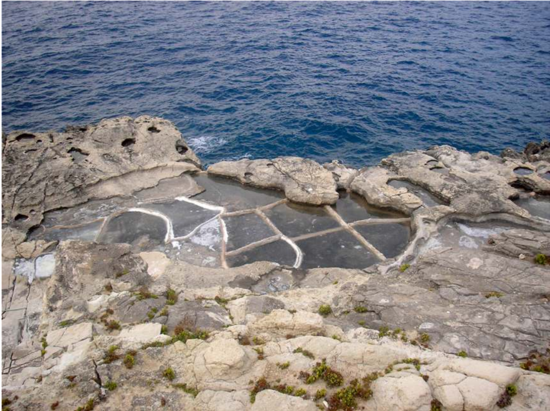
Figure 4. Kokkino Chorio (Crete): Tanks for sea salt production made of rock and cement (photo taken by the author).
