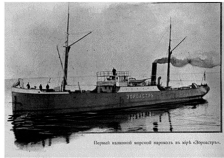
Figure 4. The world’s first oil sea tanker, “Zoroaster.” Source: The Thirty-Five Years of Activity of the Association of the Oil Production of the Brothers Nobel. 1879 – 1909, p. 150.
