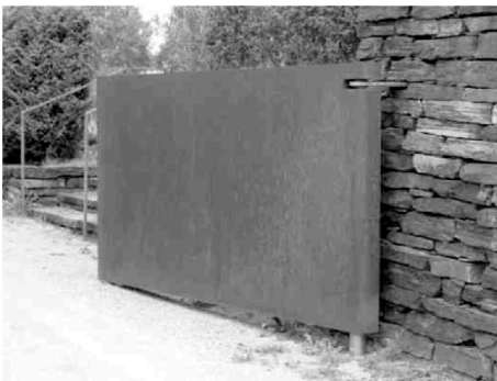
Figure 2. Andreas Meck, Stephan Köppel, funeral hall, Munich (Riem), Germany, 2001 (detail). Photo by author.
