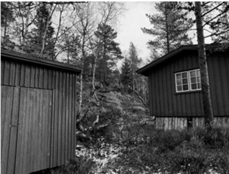
Figure 2. Norwegian cabin in Storeblevegen 433, 3680 Notodden – detail view from outside bathroom/storage space (left) and main construction. Source: author, 2021.
