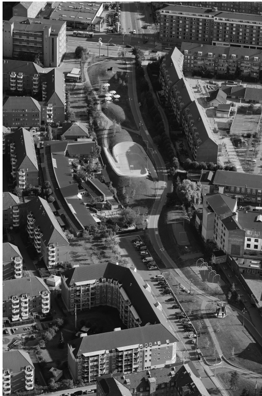
Figure 6.1 Superkilen , 2012. Urban park in Copenhagen. Den grønne park (‘The Green Park’). Commissioned by the City of Copenhagen and Realdania. Developed by Superflex in close collaboration with Bjarke Ingels Group (BIG) and Topotek 1. Photograph: Iwan Baan.
