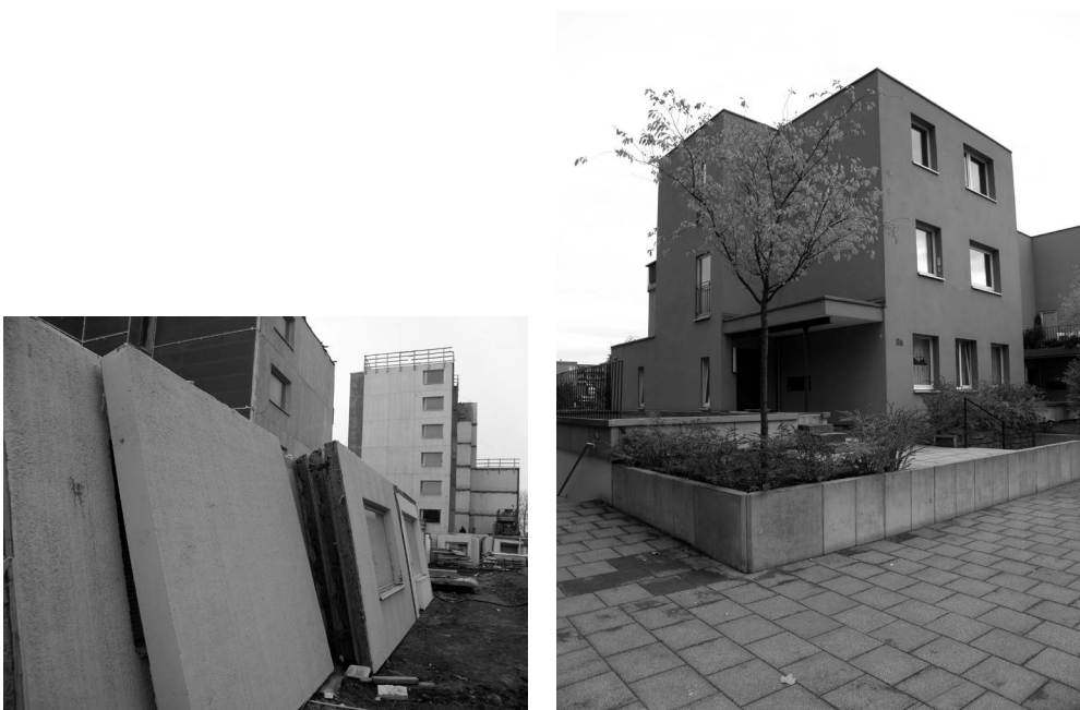
Figure 3.1 Concrete elements deconstructed from the buildings behind them (left). Location: Finland. A new building made from deconstructed elements (right). Location: Germany. Photos: SH.
