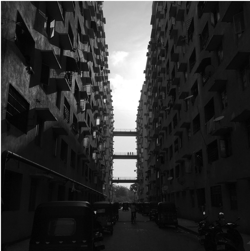
Fig. 8.4 New UDA housing development
