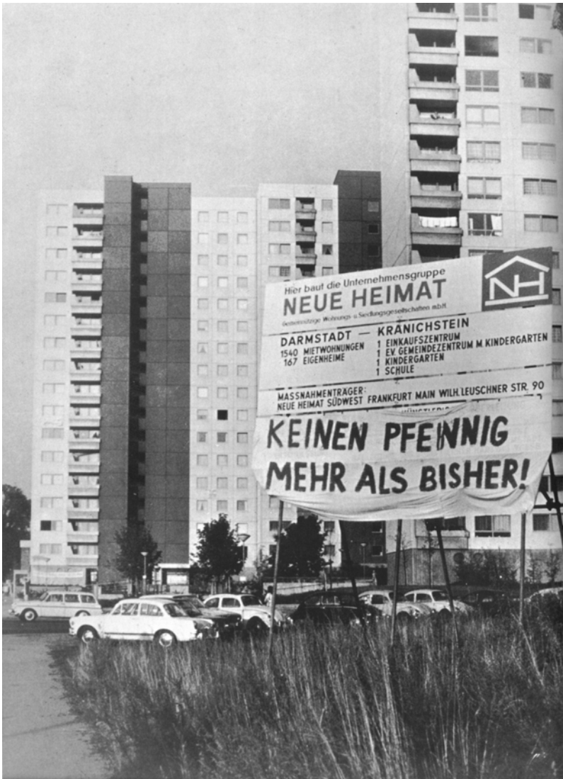
Figure 31.5 “No Penny more as before!” Large-scale housing estate Darmstadt Kranichstein, 1970.
