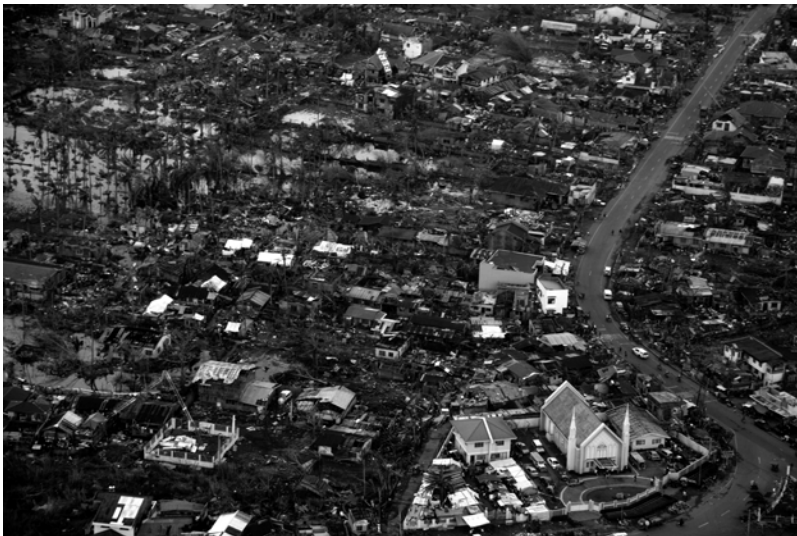
Figure 33.1 Sudden and large-scale flooding and building destruction following Typhoon Haiyan, Tacloban, the Philippines.
