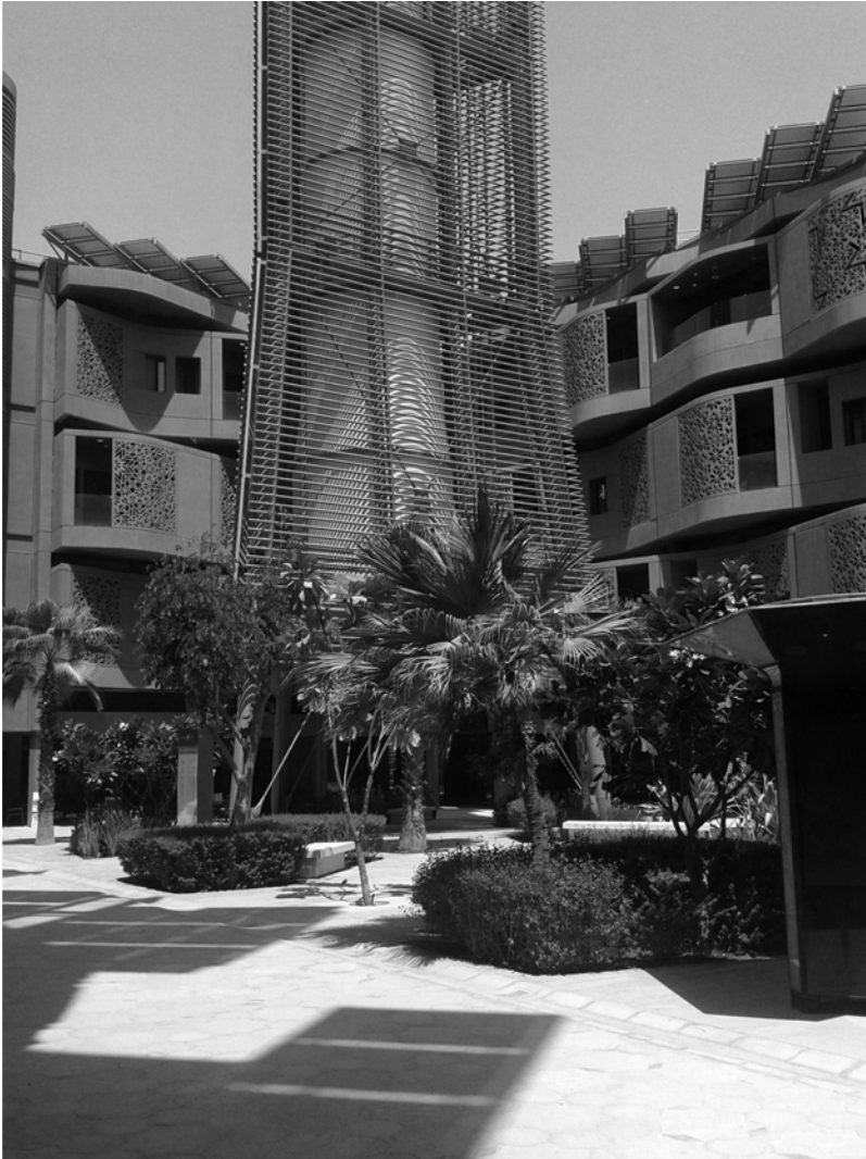
Figure 21.4 A view of the central square of Masdar City (Abu Dhabi), with its wind cooling tower, planted and shaded public space, solar-protected architecture, and photovoltaic solar panels on the roof.
