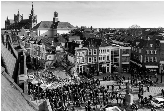
Photo 8.2 The collapsed building next door to the former house and studio of Bosch (photo: Marc Bolsius).
