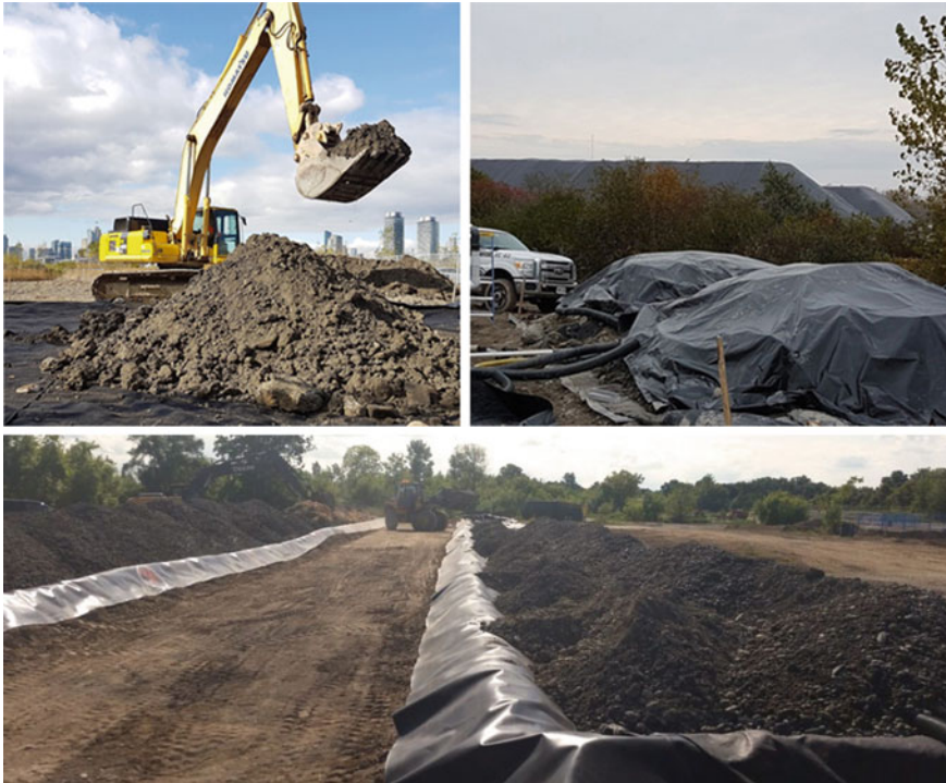
Fig. 14.6 Ex situ bioremediation—enhanced bioremediation of PHC in biopiles. The most common application is to treat soils contaminated with PHCs by adding nutrients, moisture, and oxygen to the soil. Photos courtesy of Vertex Environmental Inc
