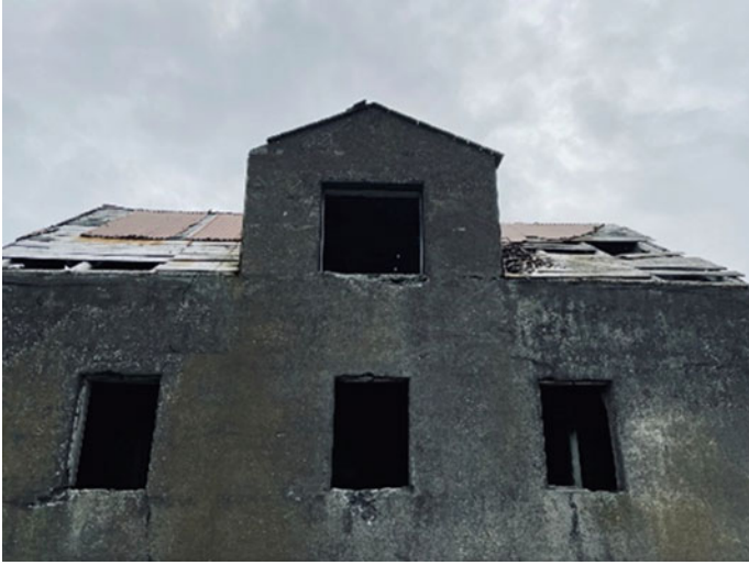
Fig. 3.14 Lichen-covered concrete wall at Rif (Photo by Katrín Anna Lund)
