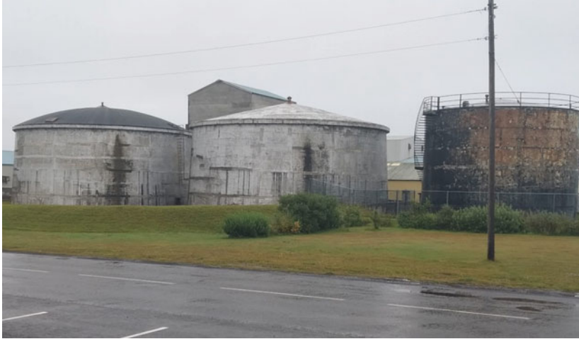
Fig. 2.3 The silos in 2020. The metal tank on the right has now been removed (Photo by Gunnar Thór Jóhannesson)
