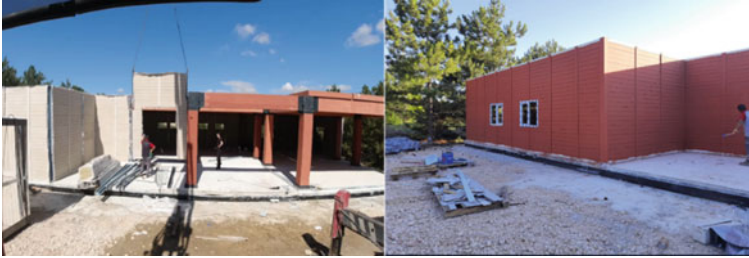
Fig. 14.10 Installation of non-structural elements
