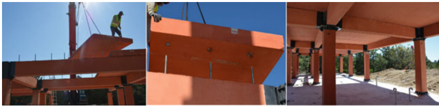
Fig. 14.9 Installation of slabs
