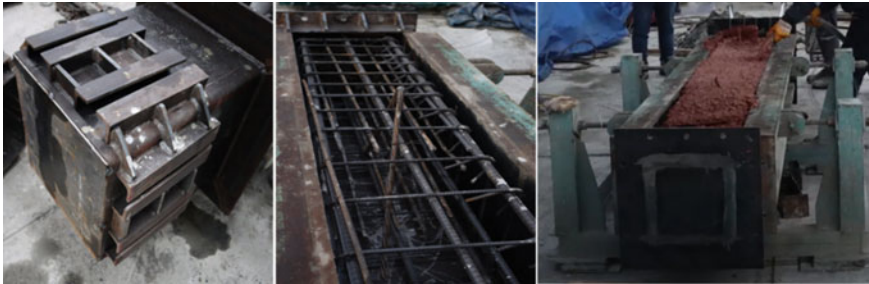
Fig. 14.6 Preparation of prefabricated geopolymer structural elements
