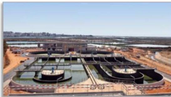
Full-scale WWTP Faro NW (Águas do Algarve, S.A.) 5000 m 3 /d, AS system oxidation ditch
