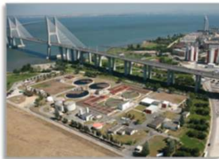
Full-scale WWTP Beirolas (Águas Tejo Atlântico, S.A.) 50000 m 3 /d, AS system A2O (Rosa et al. 2019)
