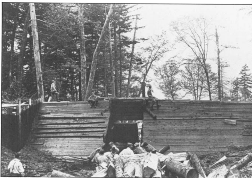
Construction of Splash Dam in Pisgah National Forest.
