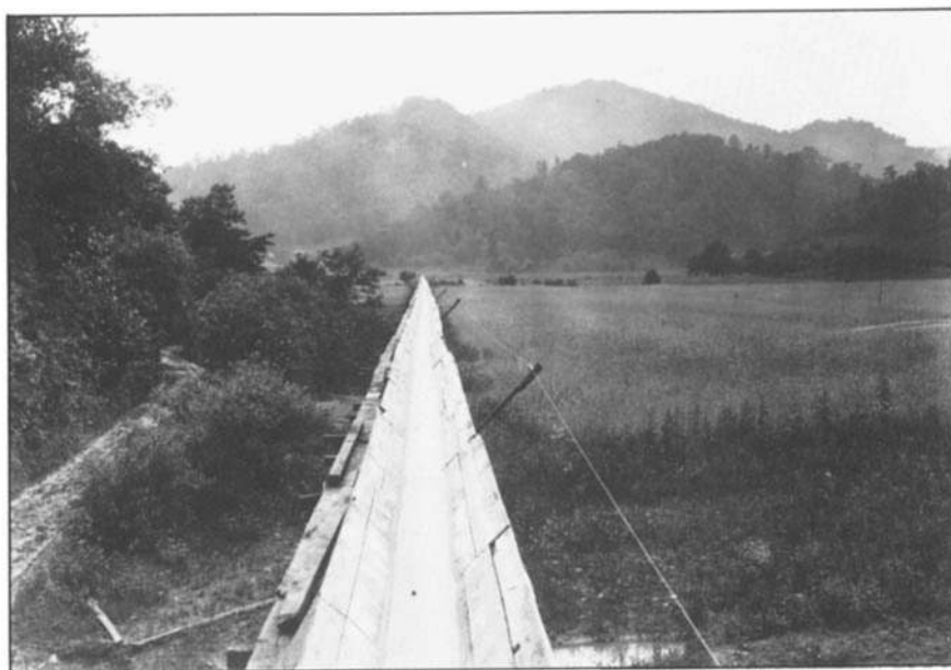
Overland, log flume on Curtis Creek, McDowell County, NC. The flume was the least destructive method for moving timber from the upper slopes to the mill site.
