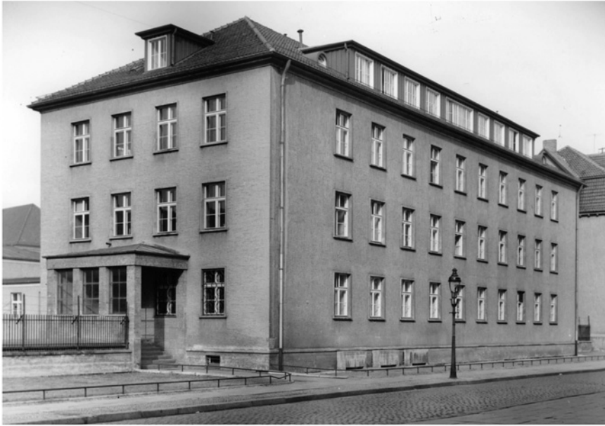
ILLUSTRATION 4 The Max Planck Institute for Physics in Göttingen on Bunsenstrasse, housed since the summer of 1946 in Building No. 10 of the Aerodynamics Research Institute (AVA), which formerly contained a cooling tunnel.
