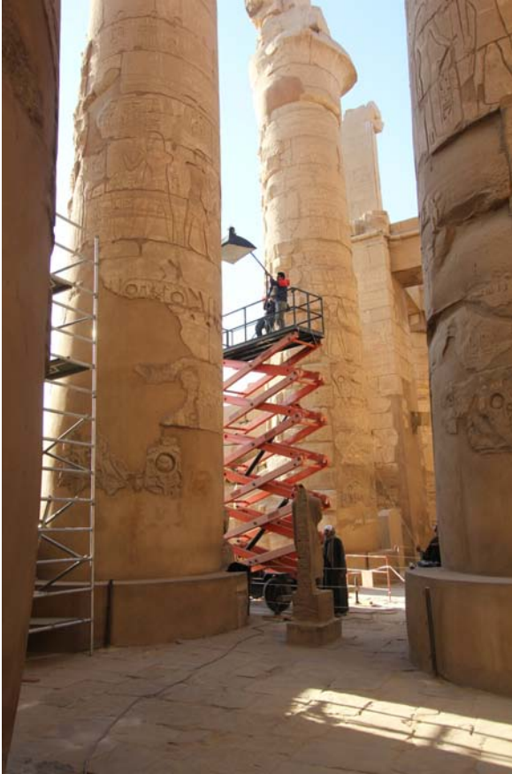
FIGURE 18.18 Scaffolding and Scissor Lift used by the project (E. Laroze)
