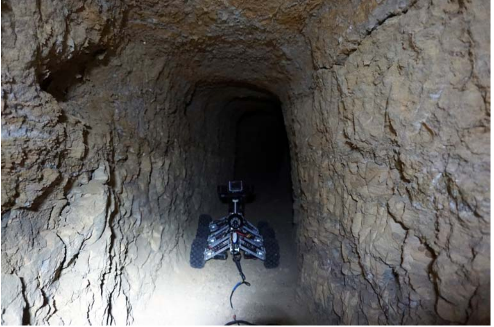
FIGURE 9.5 Southwest Roadside 10, 27 meter long tunnel
