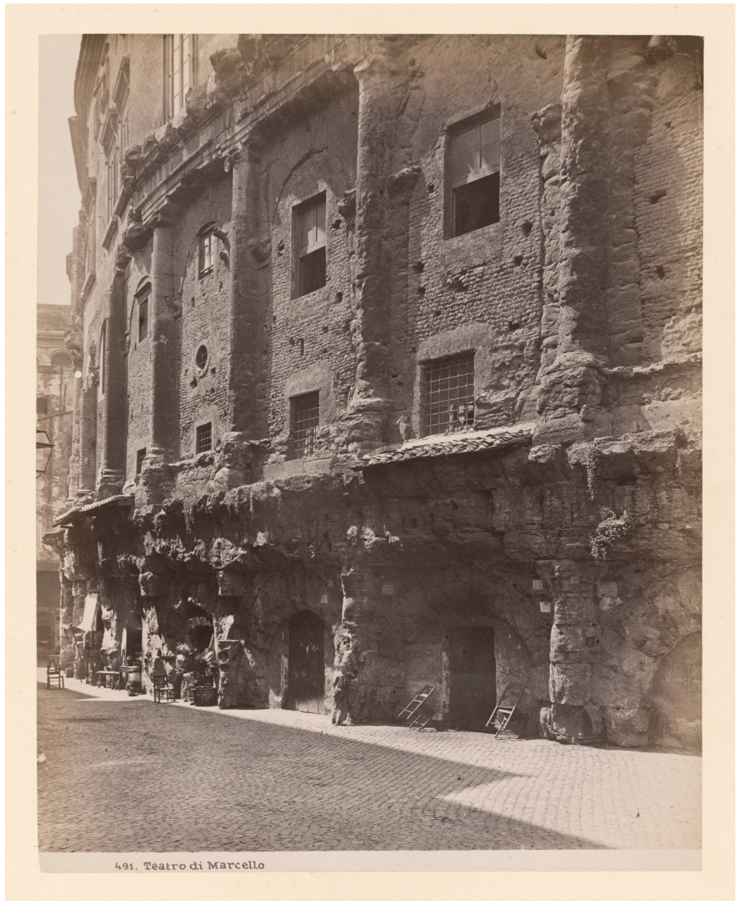
Fig. 1. Photography of the Theatre of Marcellus occupied by shops (1930s).
