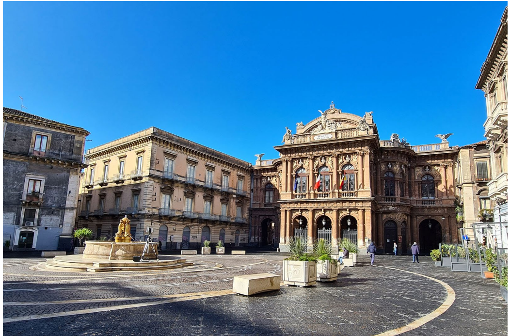
Fig. 1. Exterior view of the Teatro Massimo Bellini in Catania. Photograph by the author.
