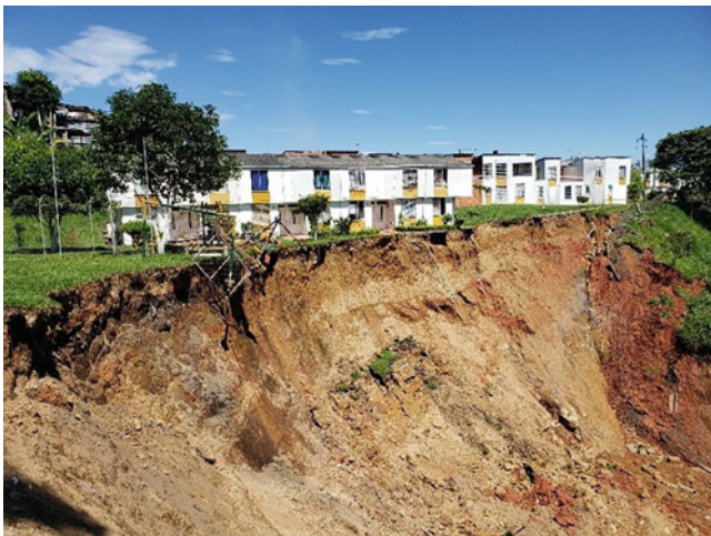
Fig. 9 Landslide principal scarp on Jun 11, 2019
