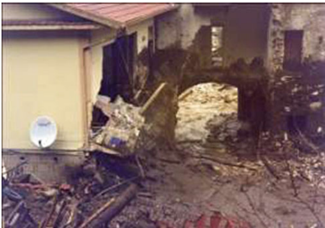
Fig. 2 Example of a building partially destroyed by a flow-like landslide occurred in the Cervinara area, Campania, southern Italy, 1999 (from Cascini et al. 2011)
