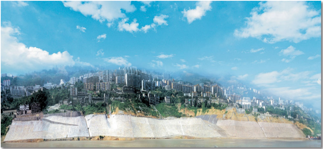
Fig. A.12 Photo of old Badong County, showing the populated area built on the Huangtupo landslide (Tang et al., 2015a)
