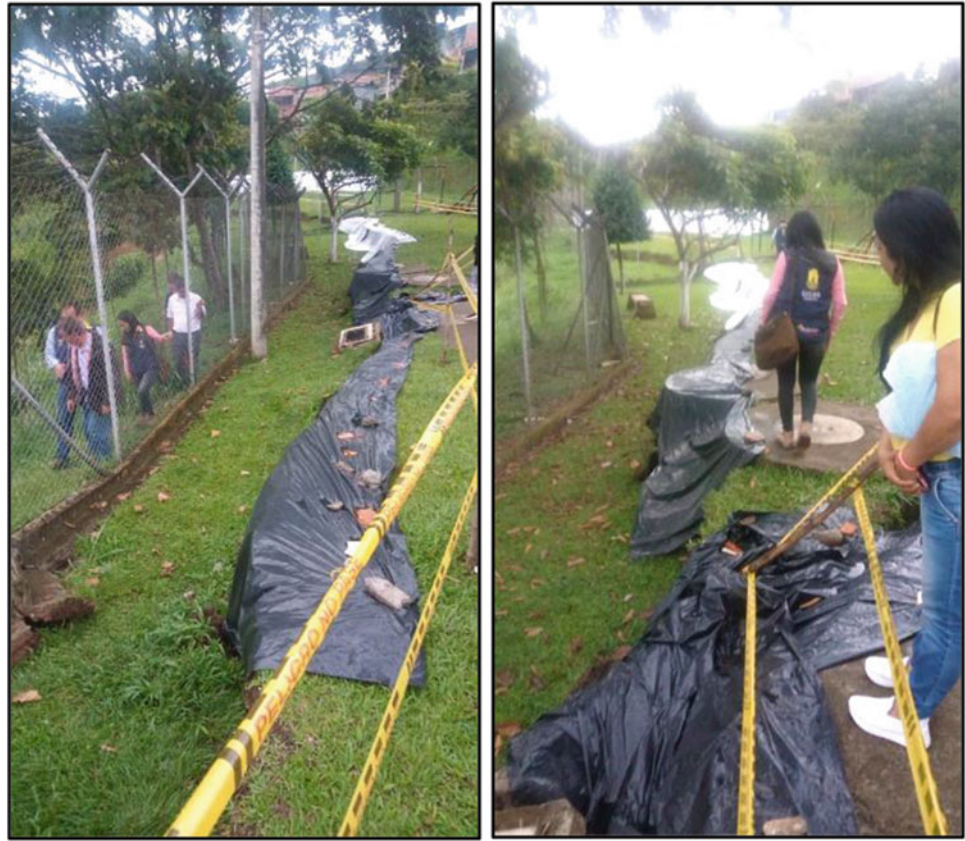
Fig. 8 Scarp evidence one day before landslide 2019
