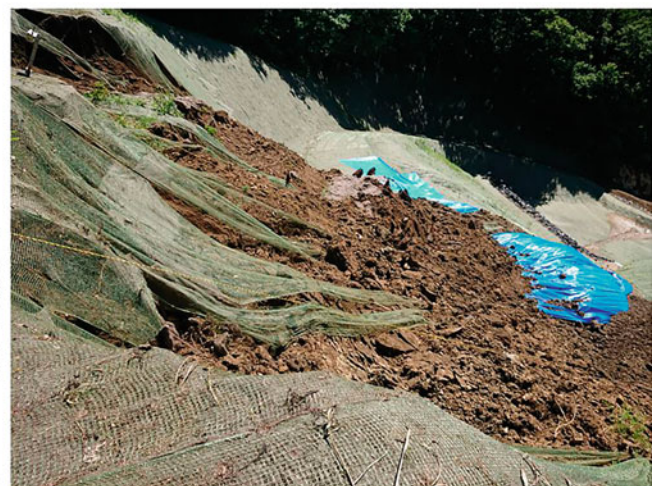
Fig. 7 Monitoring at landfill slope in Tokyo. (a) Plan view and tilt sensor locations. (b) Appearance of slope failure
