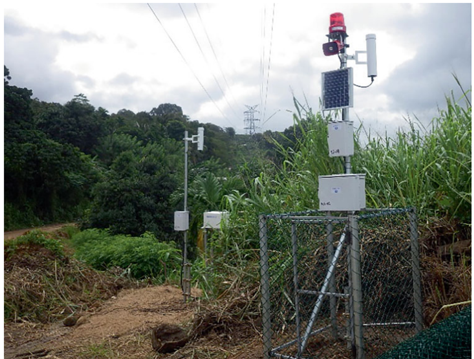
Fig. A.44 Compact alarm device to alert local people to landslide risk
