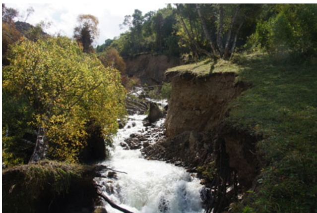
Fig. 7 New Gerkhozhan-Su River channel (Photo of O.V. Zerkal)
