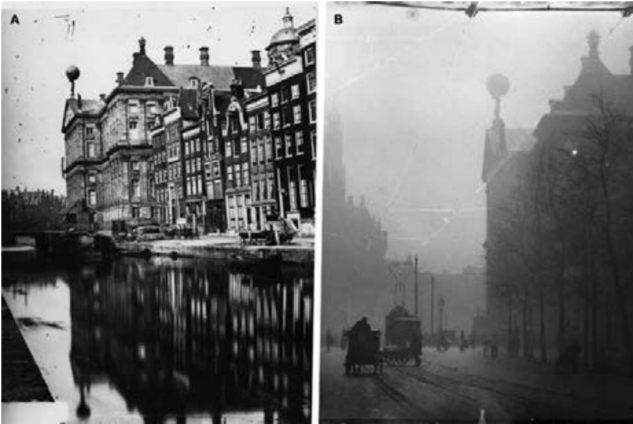
Figure 2.1. The canal along the Nieuwezijds Voorburgwal in Amsterdam had been dug in the fifteenth century and was drained in 1884 to accommodate traffic and the transportation of goods. As a consequence, the figure of Atlas, located on the roof of the royal palace, overlooked not (A) silent water but (B) bustling traffic.
