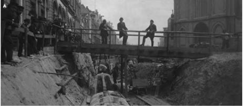
Figure 2.2. (A) The draining of canals opened up the possibility of implementing new technologies underneath the city's skin. Here a sewage system was installed on the Nieuwezijds Voorburgwal in 1884. (B) Berlage and his peers introduced modern, straight streets to Amsterdam. This image shows the Hoofdweg in 1920.
