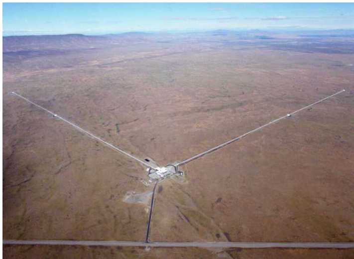
Figure 1.2.9: A LIGO gravitational wave detector. An aerial photograph of one of the two gravitational wave interferometers. A laser beam gets split after which the beams travel forth and back through two orthogonal legs. If a gravitational wave passes through one of them, the two signals show a detectable phase difference after returning. (Source: Advanced LIGO)
