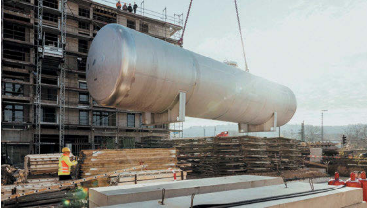
Figure 9.6: The hydrogen tank is lowered into the underground energy center. (Source: Maximilian Kamps, Agentur Blumberg GmbH)
