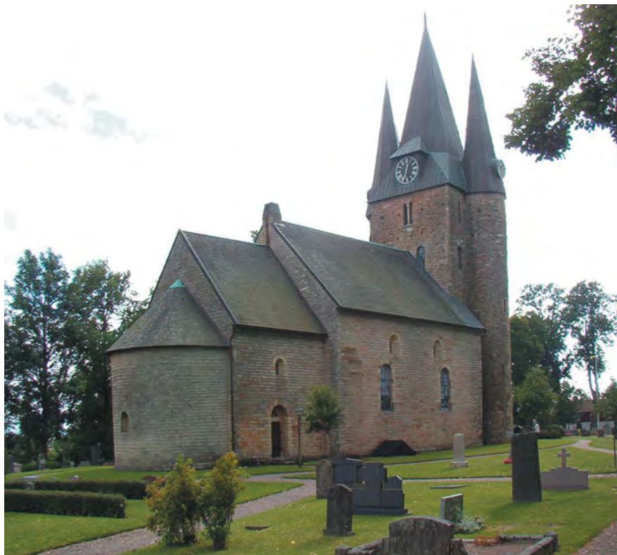
Fig. 11: Husaby Church (early twelfth century), Västergötland, Sweden. On the floor above the ground level in the western tower there was an opening towards the nave. Next to it were holes for beams which carried a balcony facing east towards the altar. Image in its original state by Fred J., licensed under https://creativecommons.org/licenses/by-sa/1.0/ .
