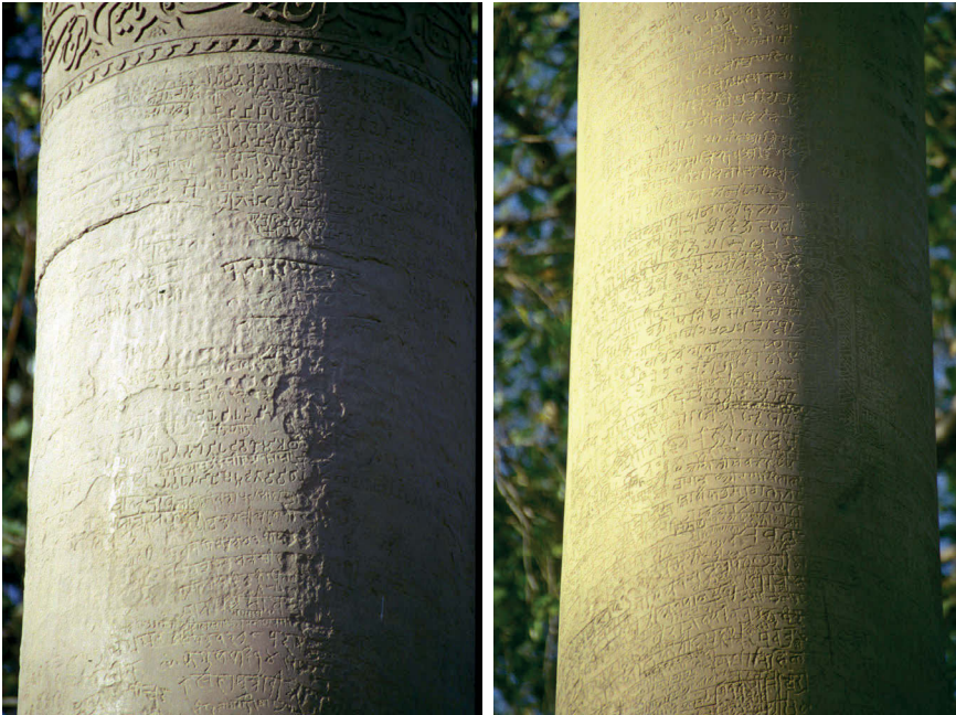
Figs 8–9: The Allāhābād pillar covered with graffiti; on Fig. 8 (left) the inscription of Jahāngīr on the top; below remains of the Aśokan edicts with interlinear graffiti; photographs courtesy Harry Falk.
