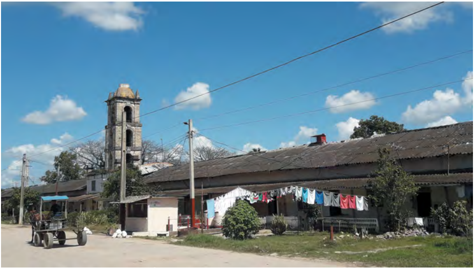
Fig. 25: The watch tower and remains of the barracones of the ingenio Álava where 781 enslaved laborers lived during the harvest of 1878–1879, 205 today the Méjico central : the museum is located to the right of the gate (photo: Ulrike Schmieder, 22.02.2019).
