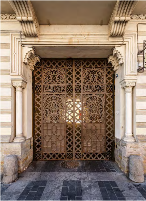
212 Muruzi House, St. Petersburg, gate to the yard, Aleksei Serebriakov, Piotr Shestov, and Nikolai Sultanov, 1874–1877.
