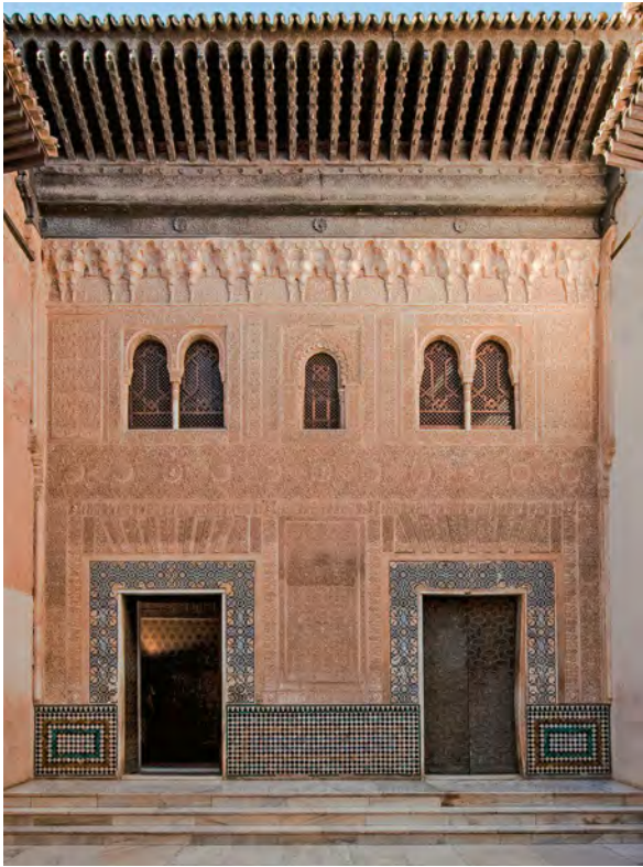
108 Alhambra, Granada, Façade of Comares, 1370.
