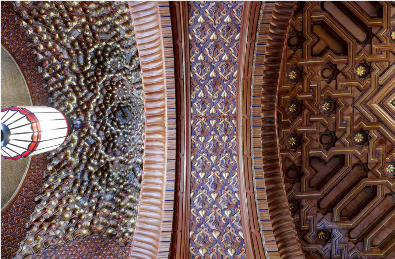
196 Villa of Franz San-Galli, St. Petersburg, muqarnaş vault and ceiling in the neo-Moorish cabinet, Karl Rakhau, 1869–1872.
