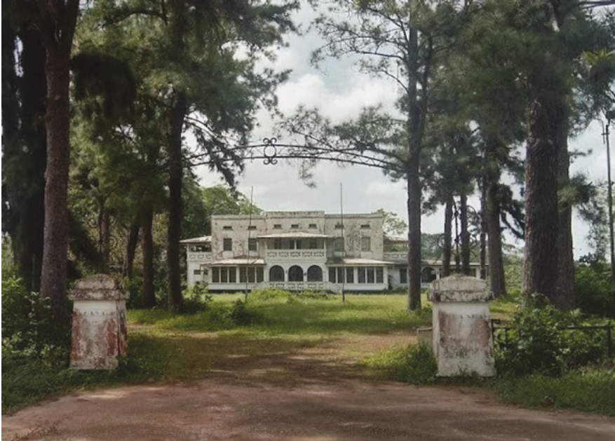
FIGURE 6.2.2 The Casa Blanca, Moengo's guesthouse, pictured in 2020 in a state of disrepair SOURCE: AUTHOR, 2020
