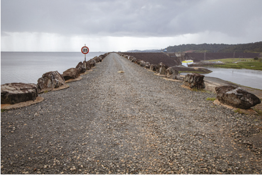
FIGURE 6.4 The Brokopondo Dam SOURCE: AUTHOR, 2020
