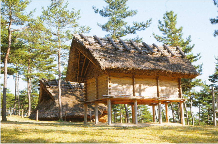
FIGURE 65 A granary from the protohistoric Kofun period reconstructed in the Miyoshi Fudoki-no-oka Park. Hiroshima-ken, Miyoshi-shi PHOTO GAUDENZ DOMENIG, 1981
