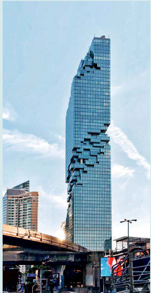
3 – THE MAHANAKHON TOWER by Ole Scheeren, 2018, in Silom Central Business District of Bangkok, Thailand
