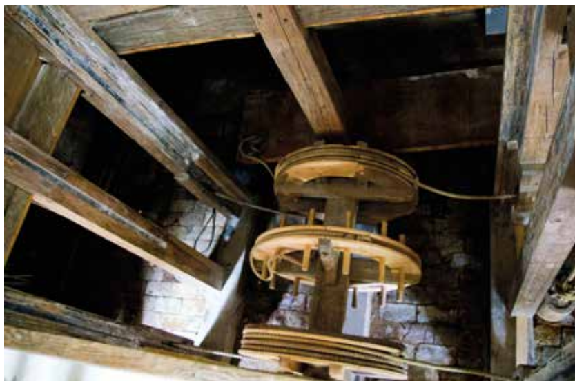
5.3 Table hoist, c. 18 th century, Confidance Room, Chinese Pavilion, Royal Palace, Stockholm. © Fabian Persson.
