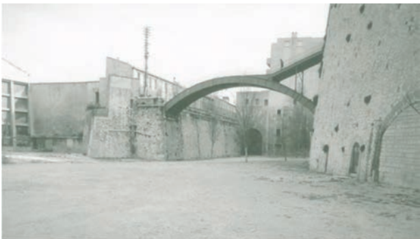
Probable ballast depot of 1824. (Photo by MTA, 1999.)
