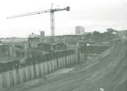
Port of Antwerp undergoing renovation. Location of the ballast depot site of 1851. Where will the seeds be moved to? (MTA, 2009.)
