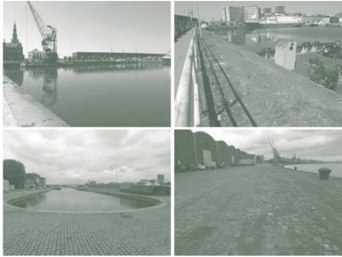
Probable ballast sites. (MTA, 2009.)
