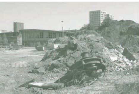
Earth being removed from the ballast depot site of 1851 in the SAS Dock during renovation works in 2009. The earth can contain seeds that arrived with ballast. Where will it begin to sprout? (MTA, 2009.)
