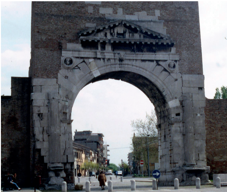
Figure 1.6 Arch of Augustus at Rimini: entrance point onto the Via Flaminia and the road to Rome. © Ray Laurence.
