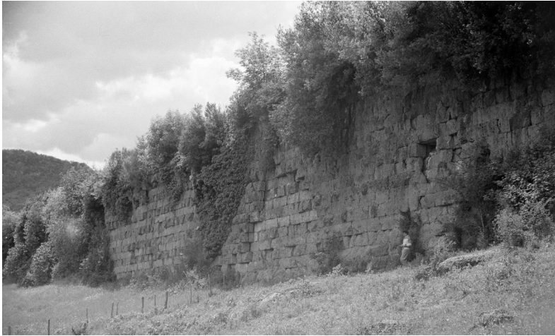
Figure 1.4 Viaduct (Muro del Peccato, Italy) carrying the Via Flaminia from a bridge across the river Treia, raising the level of the road by 45 metres to the top of the valley. Courtesy of BSR Photographic Archive, Robert Gardner Collection, rg-1524.
