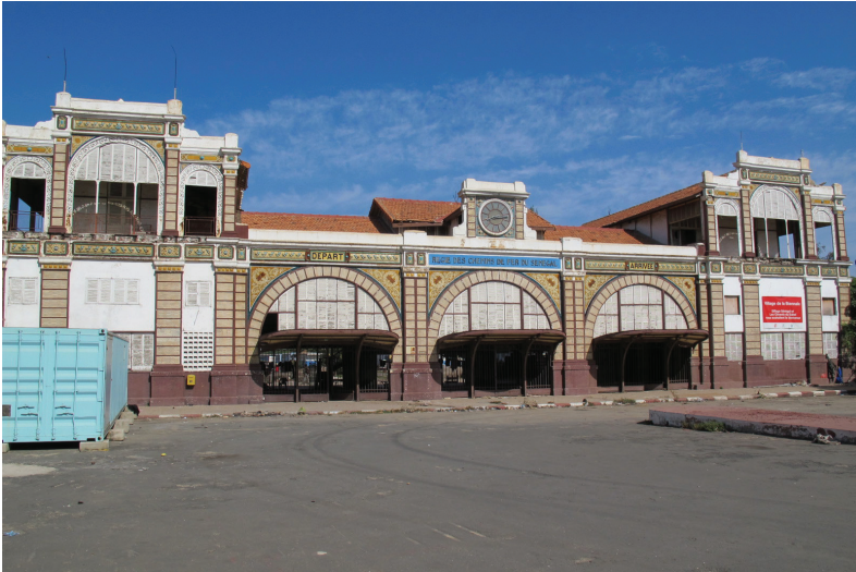
Figure 1.1 La Gare, the former terminus station of the Dakar–Niger railway in the Senegalese capital. Photo by Peter O. Jonsson, 2013.
