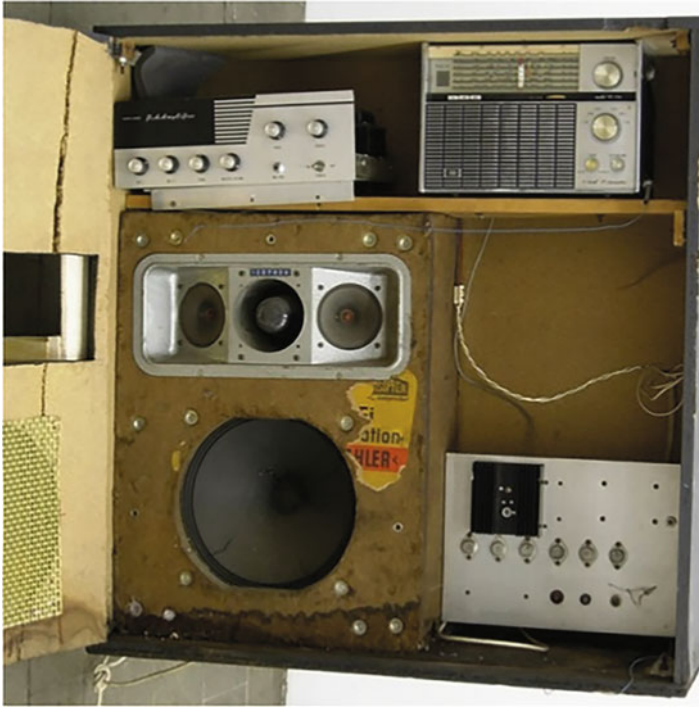
Fig. 13 Cabinet containing the audio technology shown open, condition in 2007 (Photo: A. Klusmeier © VG Bild-Kunst, Bonn 2021)
