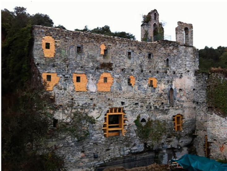
Fig. 2 Santa Catalina de Badaya (SP) restored by isuuru architects (Source: http://isuuru.com/pat_consolidacion.html . Accessed 29 Jan 2022): Restored ruin with clearly contrasted wooden additions and less visible consolidations (Photo: © isuuarquitectos)
