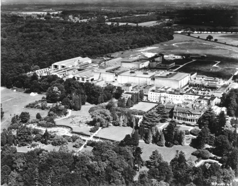
Fig. 7.1 Aerial view of Pinewood Studios, 1958. Alamy stock images
