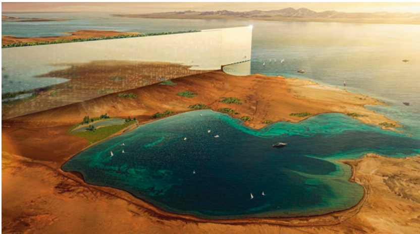
Fig. 7.1 Mockup of the Line plan. This image shows a mirrored building that is long and tall but very narrow. The mirrored surface reflects the desert and water from the ocean. (Image credit: NEOM, (2022) NEOM . Accessed November 30, 2022. ( https://www.neom.com/en-us/regions/theline ))
