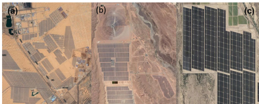
Fig. 2.4 Photovoltaic black surface in a Zhongwei, China, b Centre solar Ouarzazate, Morocco, and c Arizona, United States
