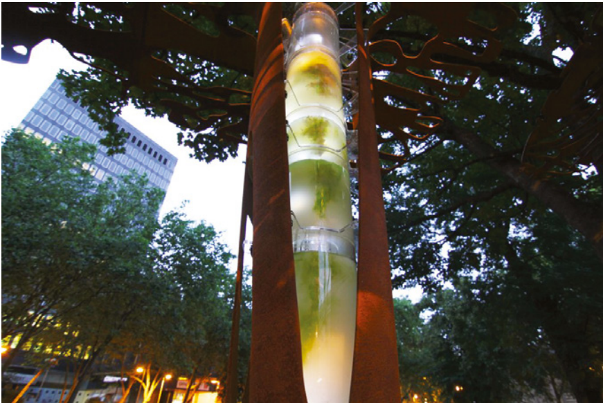
FIGURE 11.8 Alga(e)zebo – photobioreactor with multiple algae species from the surrounding embedded in double curved steel structure. Installation located at Euston Square Gardens built on the occasion of the London Olympics, 2012. Team: marcosandmarjan (Marcos Cruz and Marjan Colletti). Manufacturer: Formstaal / CSI, Stralsund Germany. Engineering: Bollinger, Grohmann und Schneider, Vienna Austria. Photobioreactor: Richard Beckett / DMC London with UCL Algae IMAGE CREDIT: MARCOS CRUZ
