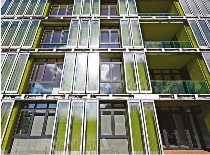
FIGURE 11.1 Solarleaf façade of B.I.Q. House with algae monoculture in flat bioreactors built on the occasion of the International Building Exhibition in Hamburg, 2013. Team: ARUP Engineering in collaboration with the Strategic Science Consult and Colt International PHOTO CREDIT: MARCOS CRUZ
