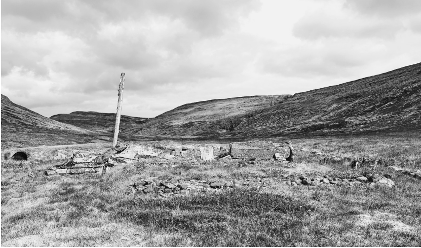
Fig. 2.26 The ruins of the farmhouse destroyed in 1948. The power of the impact of the avalanche appears to have shifted the whole upper structure of the house, whose remains are offset from its foundations by around two meters. © M. Egeler, 2019.
