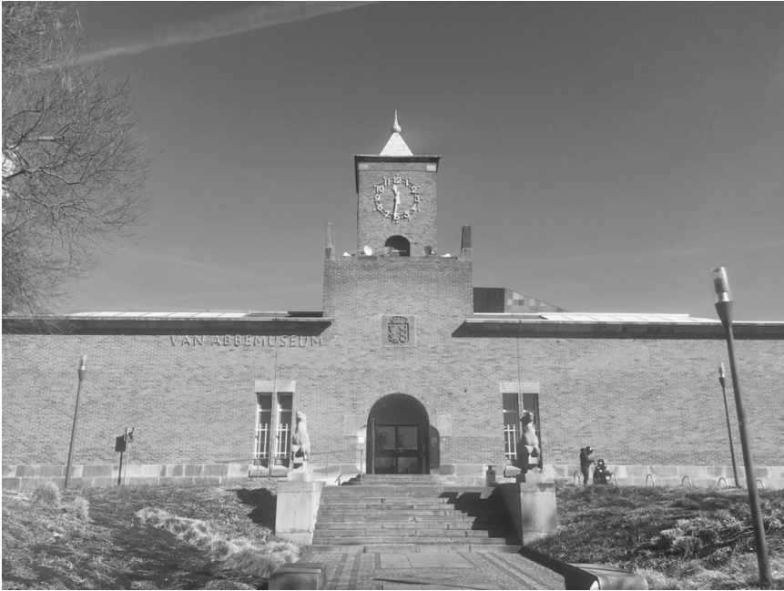
Figure 5.1 The façade of the original building with a small snippet of the 2003 addition coming above the right side of the clock tower. Photograph by the author. Used with kind permission of the Van Abbemuseum.
