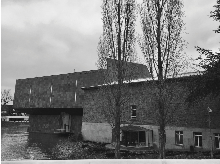
Figure 5.2 An exterior view of where the old and new buildings merge showing their situation along the River Dommel. Photograph by the author. Used with kind permission of the Van Abbemuseum.
