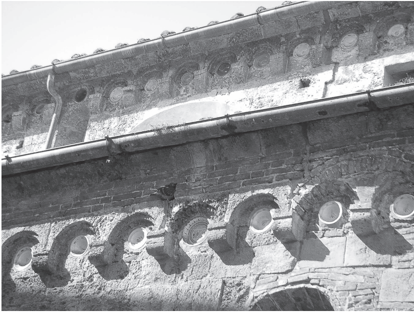
FIGURE 5.3. Lustered ceramics used as bacini, at least some from Murcia, on church of Sant'Andrea, twelfth century, Pisa. Photo: Wikimedia Commons; photo uploaded by Sailko, licensed under the Creative Commons Attribution-ShareAlike 3.0 Unported (CC BY-SA 3.0) license ( https://creativecommons.org/licenses/by-sa/3.0/ ).
