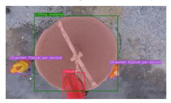
Figure 4: Illustration of worker tracking with unique identity assigned to different workers
