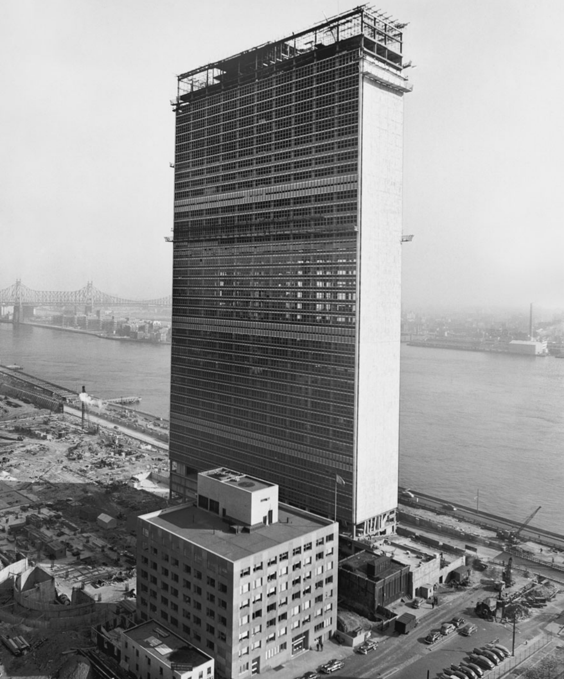
The United Nations Secretariat building under construction in 1949, when thousands gathered for the ceremony dedicating the cornerstone of the “world capital.” (William Eckenberg/ The New York Times /Redux)
