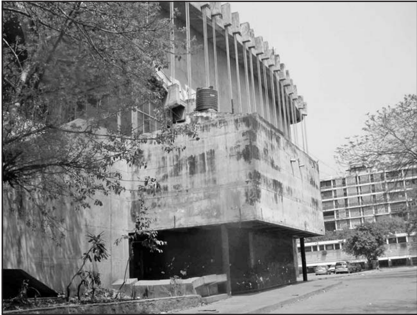
Figure 3.6. The theater's reinforced concrete construction reflects the influence of post-Le Corbusier modernism.
