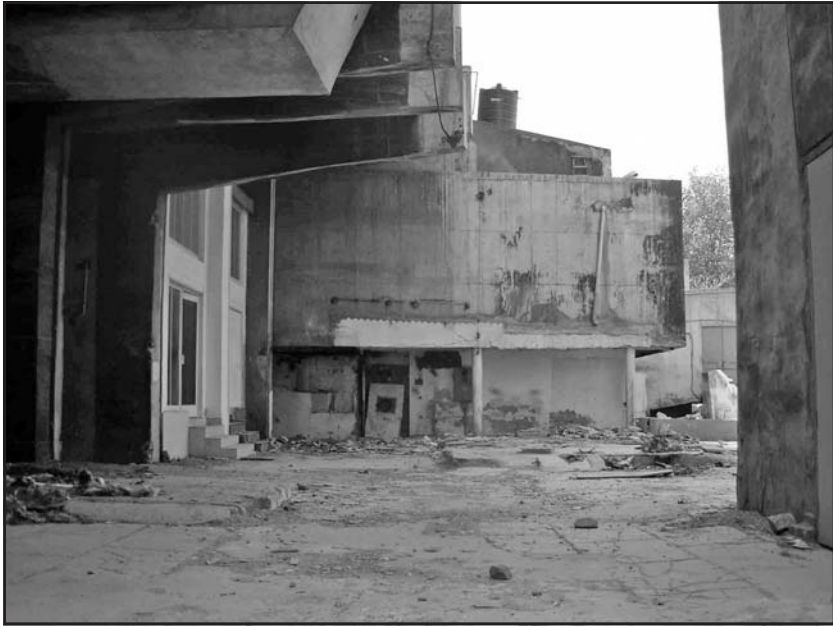
Figure 3.5. The Chanakya demolition in progress.
