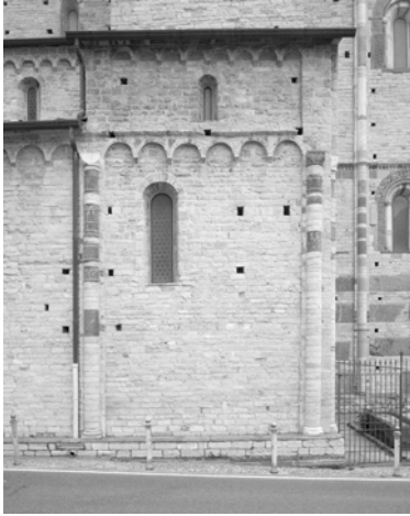
2 Basilica of Sant'Abbondio, Como, south elevation.
