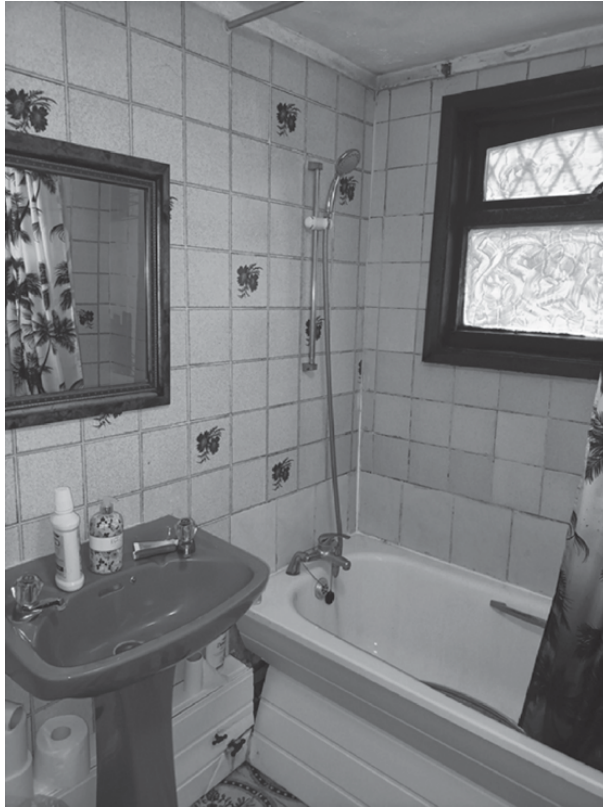
Figure 2.5: Bathroom on the ground floor, shared by tenants in Rooms 1, 3 and 4
