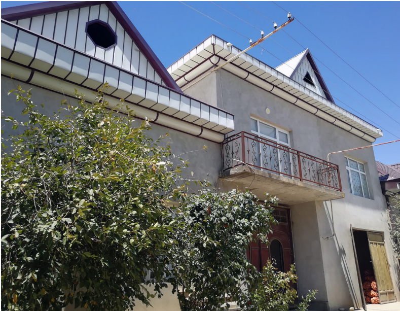
Figure 0.2 A migrant house under construction, Sughd Province, summer 2018.
