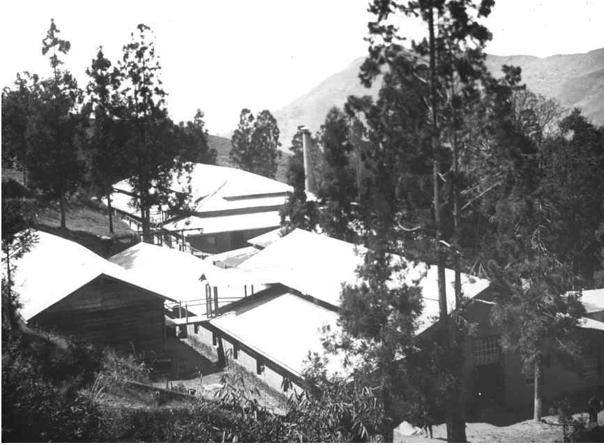
FIGURE 15. Government quinine factory at Mungpoo, exterior, ca. 1910. Credit: Lantern Slide, British Library, Photo 397 (72).
