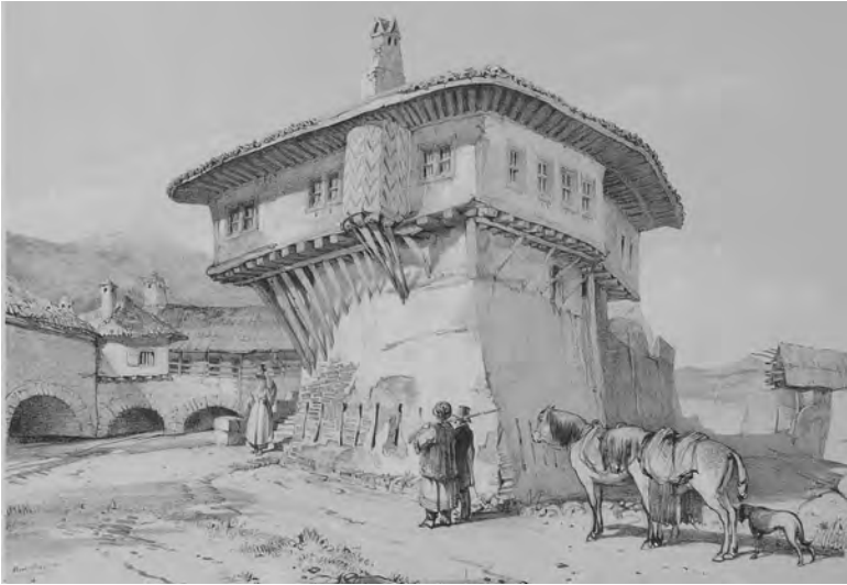
Figure 15 John Richard Coke Smyth and John Frederick Lewis, New Orsova; Exterior of the Pasha's Residence (1838).
