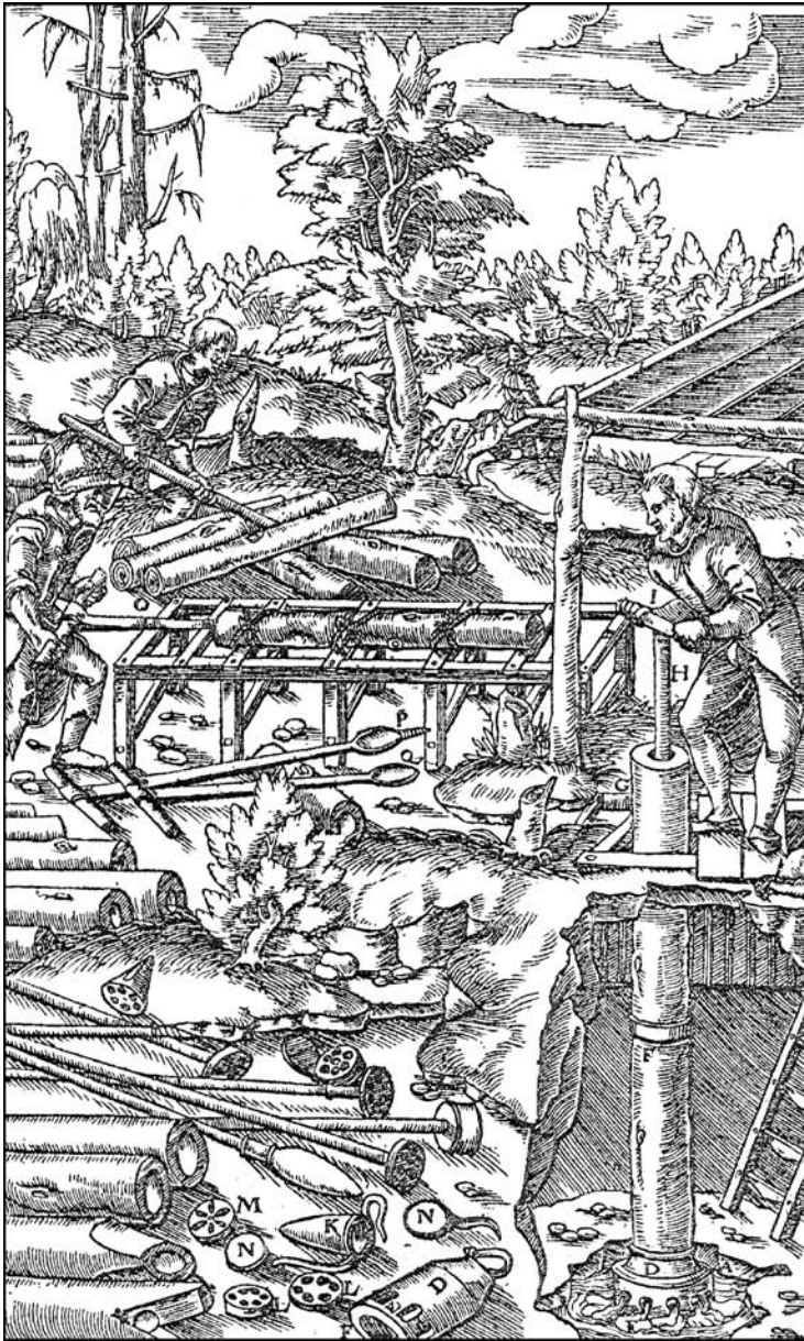
Fig. 56: Horizontal manual drilling of a pipe, mid-16 th century. P – a spoon auger with a twisted point; Q – a wider spoon auger, after: Agricola 1928, p. 148.
