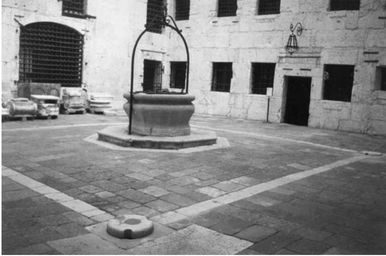
Fig. 20: Venice. Casing of a filter cistern together with four openings at the level of the pavement through which rainwater could pass. Photograph: U. Sowina.
