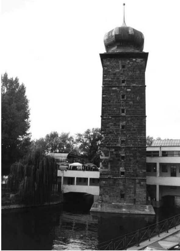
Fig. 55: Prague. The Šitkovská vodárna (water tower) in the New Town. Photograph: U. Sowina.
