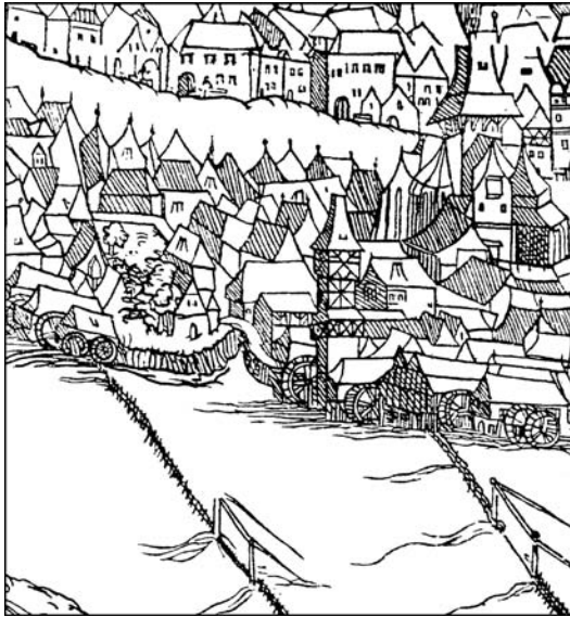
Fig. 54: Prague. The Šitkovská vodárna (water tower) with mills on the Vltava River, 1562, after: Jásek/Fiala 2004, p. 17.
