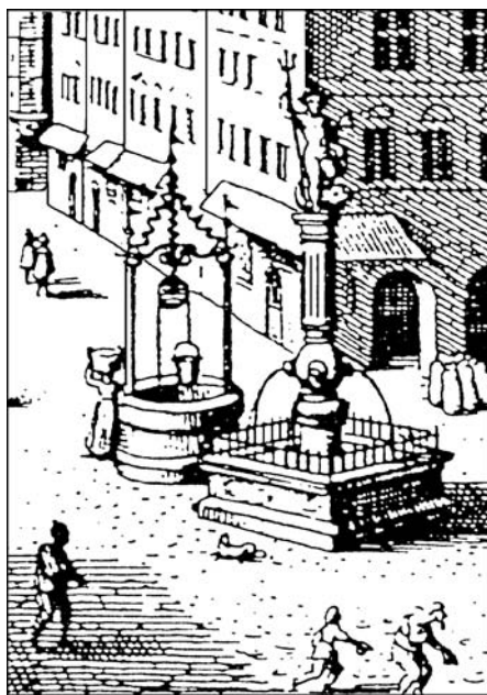
Fig. 62: A water storage reservoir next to a dug well in Marienplatz in Munich, mid-17 th century, after: Hoffmann A., 2000a, p. 34, fig. 26.
