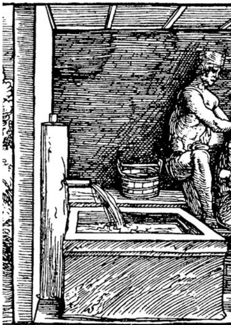
Fig. 64: A water storage reservoir connected to a water supply system – a chest with a water-pillar. Petrarch, De remediis utriusque fortunae , Augsburg 1532, after: Braudel 1992, fig. no. 3 after p. 32.
