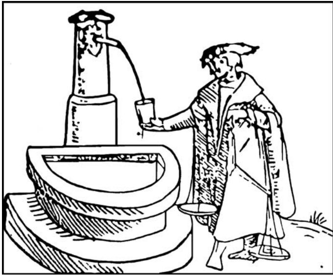
Fig. 65: A water storage reservoir connected to a water supply system – a reservoir with a water-pillar, after: Crescenzi 1548, p. 5.
