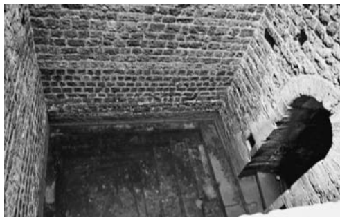
Fig. 42: Speyer on the Rhine. The interior of a mikveh built in 1126, with water from the water-bearing stratum. Photograph: A. Janeczek.
