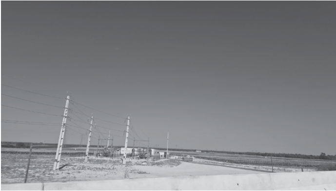
Figure 4.1: Large solar plant and transmission grid
