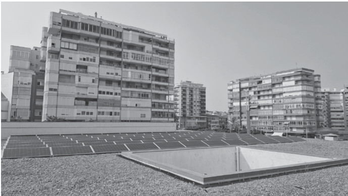
Figure 6.1: Rooftop solar plant at the Almada cultural centre
