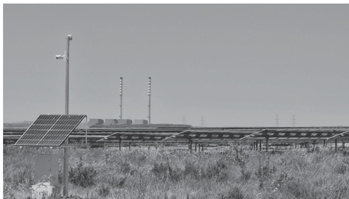
Figure 7.4: Large solar plant with the Sines coal thermal plant in the background
