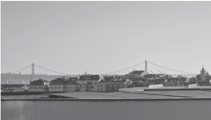
Figure 8.2: Dusty inefficient solar plant on a Lisbon restaurant
